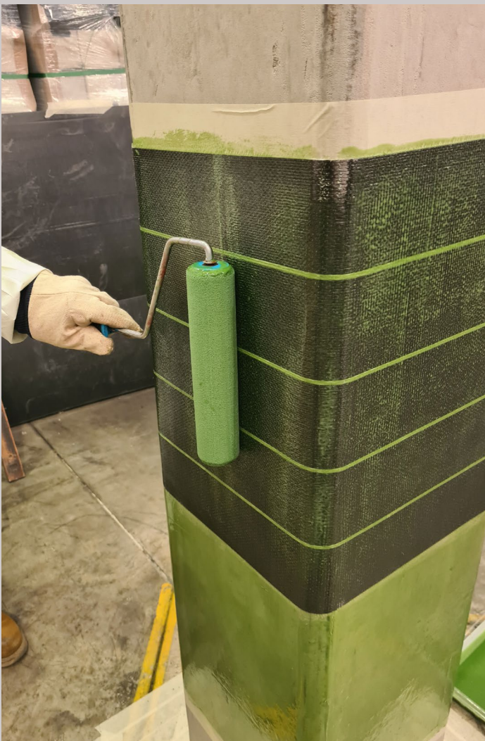
Carbon reinforcement to increase the strength of structural elements
