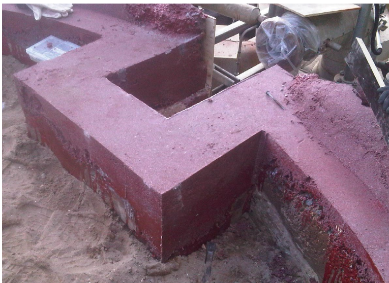
Repairs to a chemical tank base
