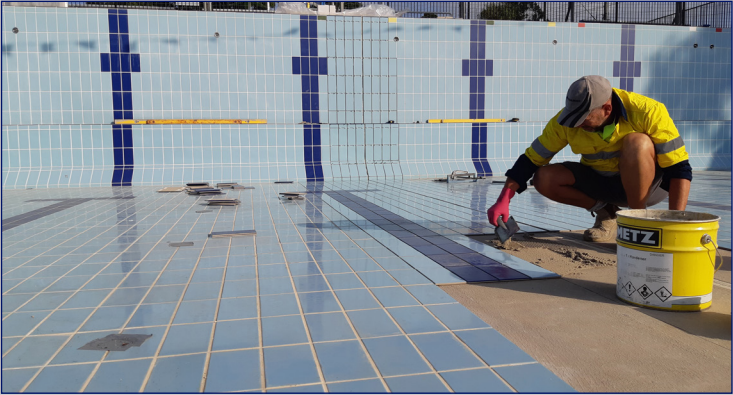
Infill tiling after installation of a properly detailed and constructed waterproofing bandage at a major construction joint.
