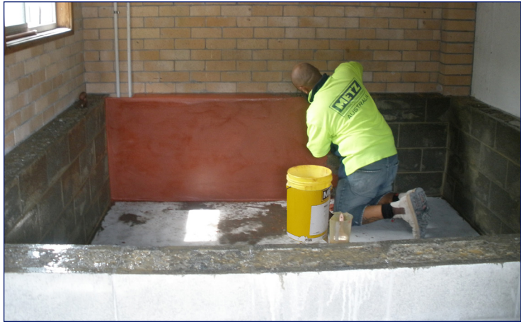
Chemical storage areas require a lining that will resist concentrated chlorine and acid. Metz manufactures a range of materials suitable for all such areas.
