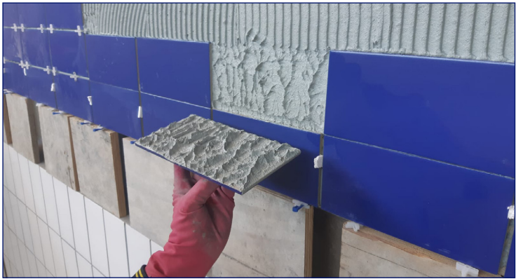
Regular quality checks are required to ensure complete adhesive coverage is obtained when tiling commercial pools. Inadequate adhesive coverage is a common contributor to tile adhesive failures Metz is called to rectify.
