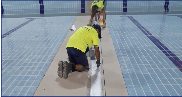
Installation of waterproofing bandage at a major construction joint. This critical work requires experience, an attention to detail and professional supervision to oversee installation.
