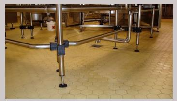
**Corrosion Resistance** - all foodstuffs are corrosive. The worst food areas are where hot fats are in frequent contact, and poultry fat is the most aggressive. All components of the flooring system must be designed to resist corrosion or the result will be impossible to clean floors firstly, thereafter unstable corroding floors not fit for purpose.
