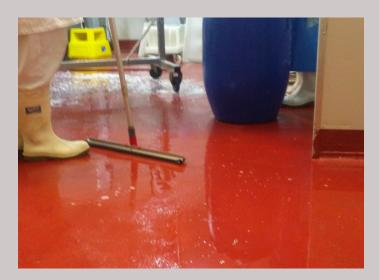
**Cleanability** - This comes from the combination of correctly installed floor slopes, an impermeable flooring material that is not overly hard to clean coupled with the right cleaning processes. Floor to wall junctions must be coved to ease cleaning.
